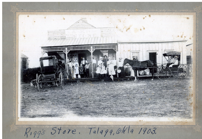
Fig. 5.17: A general store in Taloga, Oklahoma Territory, around 1903. During the first days of settlement in Taloga, members of the Dalton Gang and other outlaws are rumored to have filed land claims, using fictitious names. Farming, ranching, and oil and gas production have remained important economic drivers in western Oklahoma to the present day.
