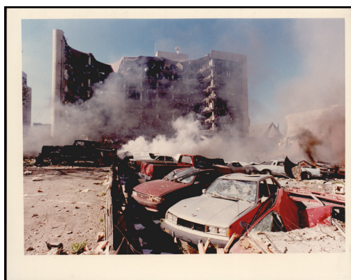
Fig. 15.2: As this photo shows, the bomb blew up the entire north side of the Murrah Federal Building and destroyed the rest of it. It also caused great damage to the surrounding buildings and area. It caused car and home alarms to go off in nearby areas as well. The force from the blast was so strong that some people reported feeling an earthquake-like sensation almost one hundred miles away.
